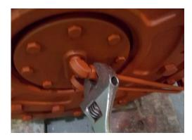
b) Screw in the nuts for the joint located at both ends of the pipe at each joint and tighten them. The pipes constitute each system of the oil feeding piping from the joint in the lower area of the motor end cover to another on top of the motor spacer as well as the oil returning piping from the joint in the upper area of the motor end cover to another in the lower area of the motor spacer. Connect the pipes cautiously not to confuse them.
