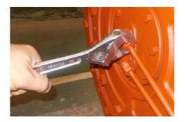
g) Attach the jacking bolts in the threaded holes at four spots on the motor jacket cover flange surface. Gradually retract the jacket cover by turning a half turn at a time of each of the four jacking bolts (following picture to the left).
